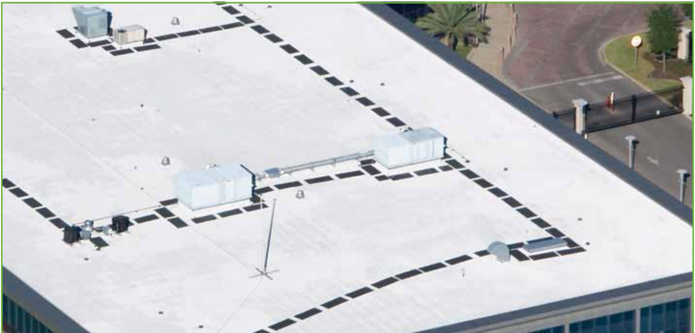
FlexGuard™ Peel & Stick™ WalkWay Pads on top of FlexWhite™ Membrane
