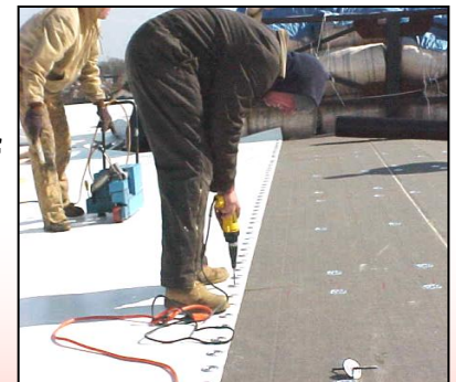
Attachment of GenFlex TPO Membrane
