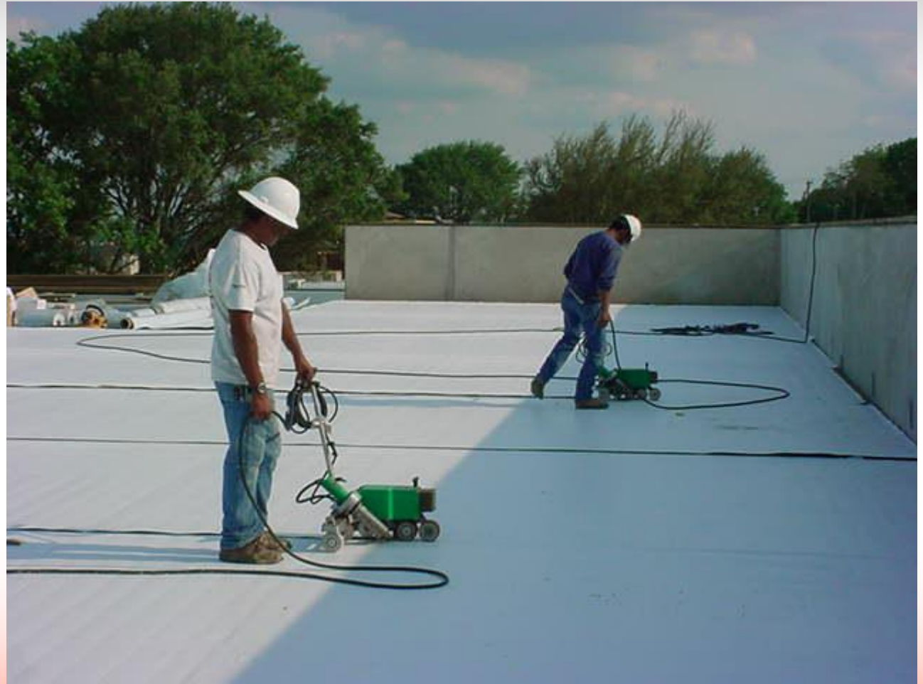
Typical Self-Propelled Hot air Welder ("Robot")
