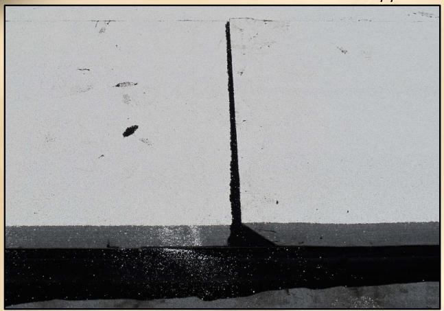
Allow for some bleed out at the side and end laps to ensure that the laps are properly sealed.
