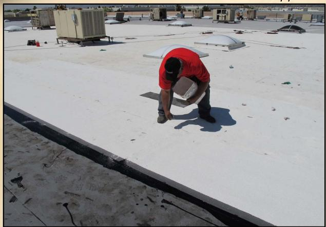
• Casting granules into the exposed LiquiGard™ is an option that offers a clean, finished look.
