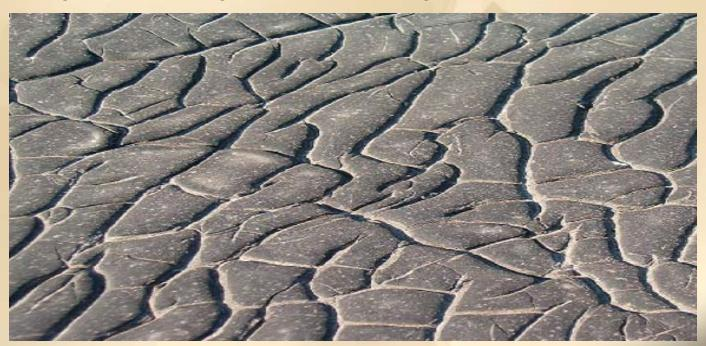
Left unattended, cracks and splits eventually develop. Water will pierce the roofing system and cause undetected damage in the roof system. As the surfacing layer fails, the fiberglass reinforcement underneath is exposed and becomes brittle. Membrane failure inescapably follows
