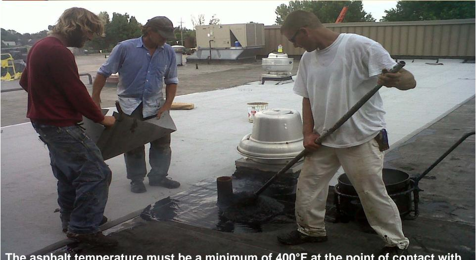
The asphalt temperature must be a minimum of 400°F at the point of contact with the membrane. Asphalt must be type III or IV or Firestone SEBS asphalt.
