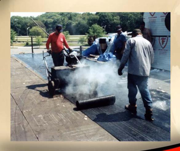
Hot asphalt is the adhesive and the waterproofing between Built-Up Roofing layers (plies)
