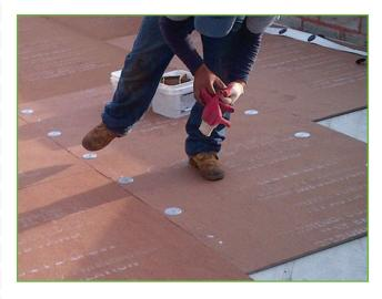
STRUCTODEK with Primed Red Coating is a highdensity, <sup>1</sup>/<sub>2</sub>" wood fiber roof cover board. It has a proprietary, patent-pending, environmentally friendly, non-asphaltic red primer on two sides to provide superior adhesion without excess adhesive absorption.
