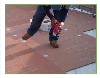
STRUCTODEK with Primed Red Coating is a high-density, ½" wood fiber roof cover board. It has a proprietary, patent-pending, environmentally friendly, non-asphaltic red primer on two sides to provide superior adhesion without excess adhesive absorption.
