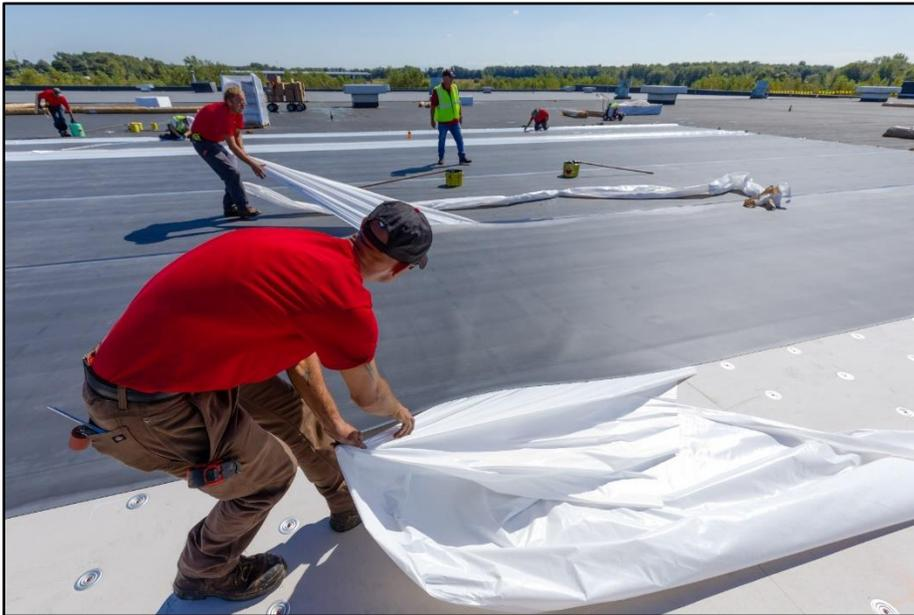
**TIP THREE:** Remove selvage edge release liner at a 45° angle, prime lap areas, and mate the seams (see Application Guide for full priming instructions). *Immediately* hand-roll the seams. Use a 1½" to 2" wide silicone roller to roll the entire seam, first at a right angle toward the outer seam edge and then along the length of the seam, making sure there is sufficient contact between membrane layers.
