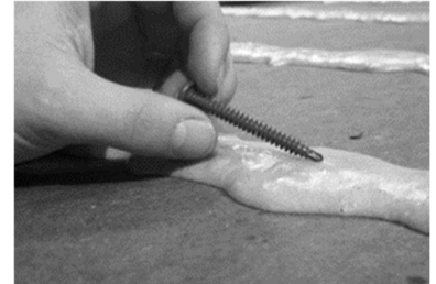
STEP 3: Tack-free stage – ready for application of EZ Fleece Backed TPO Membrane (after 5 -7 minutes)
