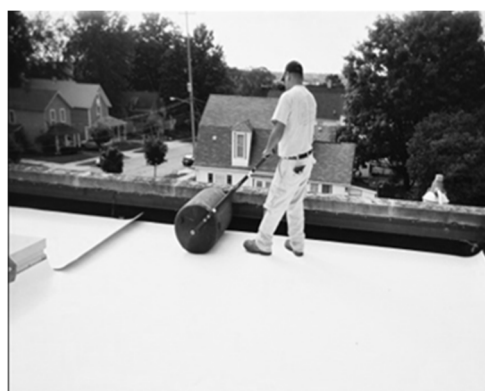
Apply pressure to the top surface of the membrane to ensure contact with a roller (not to exceed 150 lb/68 kg)
