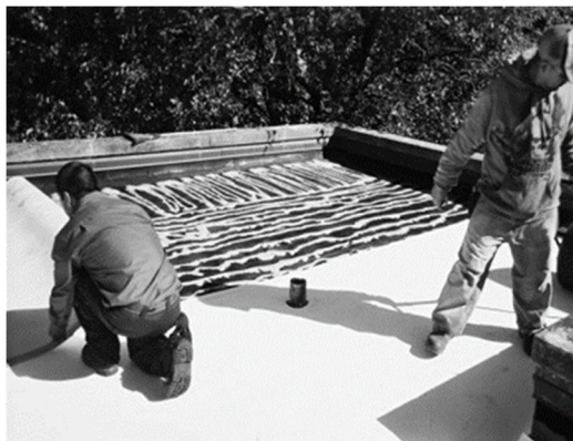
Roll EZ Fleece Backed TPO into LRF Adhesive
